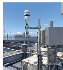
Weather sensors to collect data at various locations such as building rooftops
