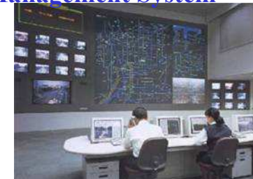
Traffic/Road Management System
