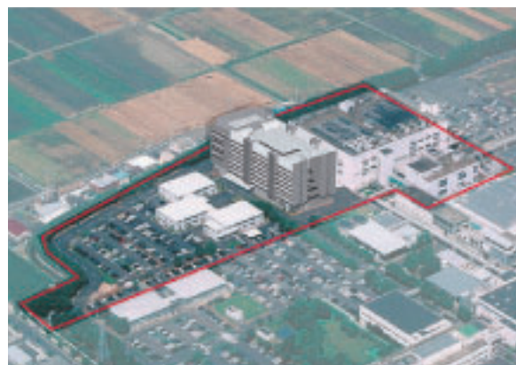
Site of the Yasu Facility and a planned new building
