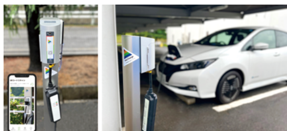
EV charging smart plug module (top) installed in an EV charging outlet to provide an EV charging and billing service
