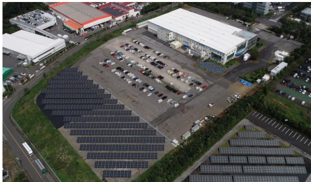
PV power generation system installed for Yamaichi Electronics
