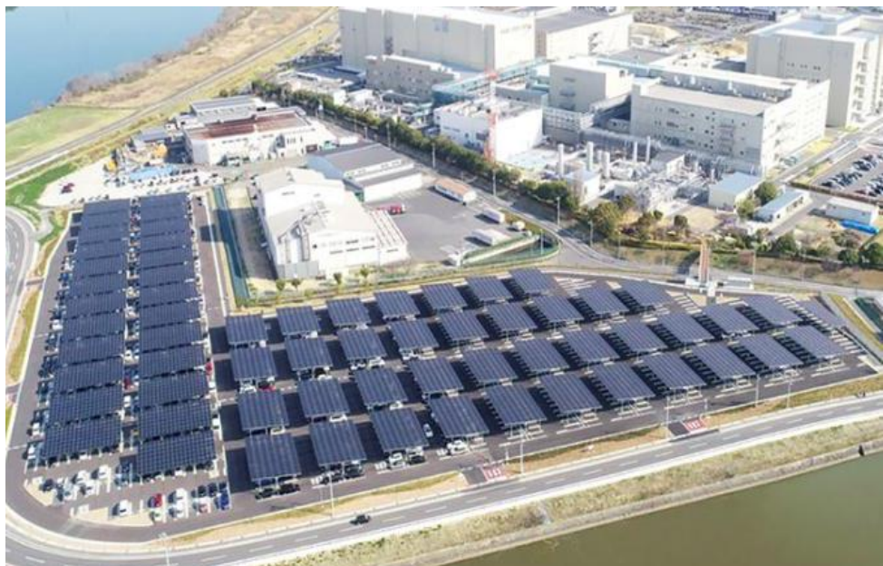
PV power generation system installed in parking lot for 1,200 vehicles
