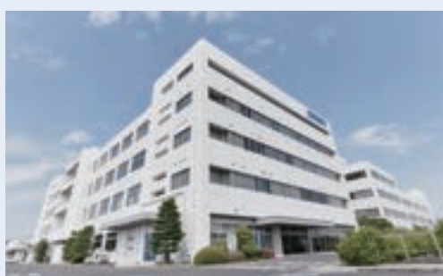
Kusatsu Plant (Exterior)
